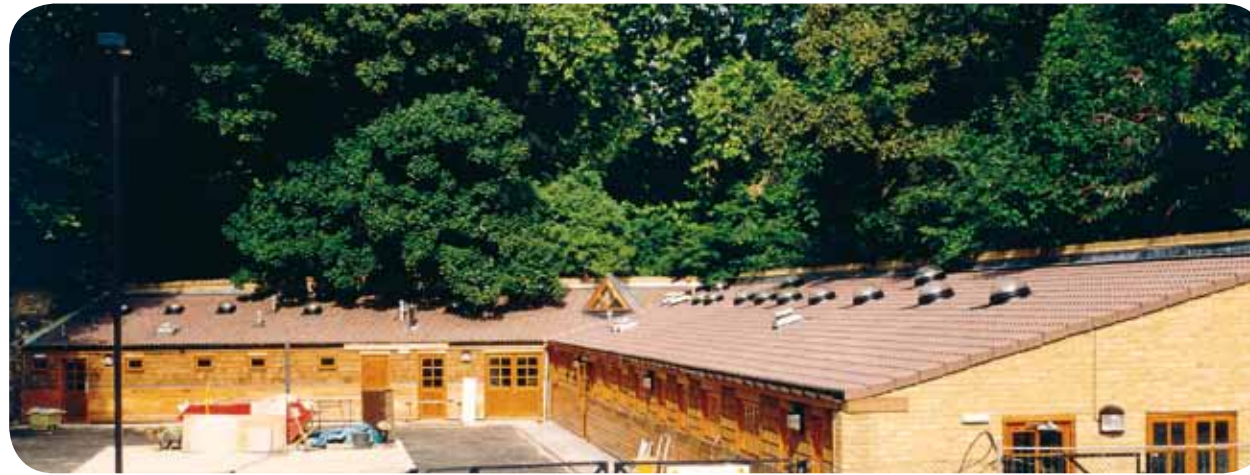
Top: Battersea Park Police Headquarters, where 19 No. 530mm diameter SUNPIPE natural daylight systems were installed to internal cells, corridors and interview rooms.
