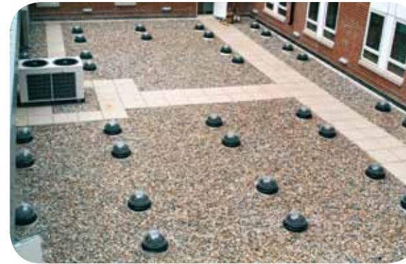
Top: Battersea Park Police Headquarters, where 19 No. 530mm diameter SUNPIPE natural daylight systems were installed to internal cells, corridors and interview rooms.
