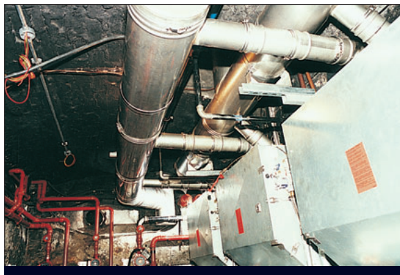
Left Supra inlet and exhaust manifolds used for a number of fully condensing boilers.
