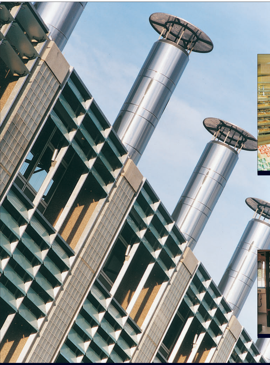
Above Europa used as a fire rated passive ventilation system at the Building Research Establishment's new Environmental Building.
