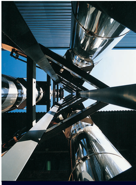
Worms eye view of the trio of SM W chimneys supported on a triangular frame.
